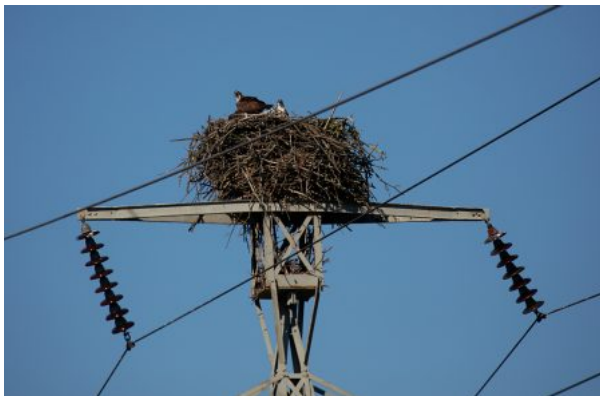
Fig. 2: Power line nest. Birds responded to the emergence of electrical infrastructure in the nineteenth and twentieth century by building their nests on top of poles and pylons. Some even dismantled wires and cables for metallic nesting material. Today, specialized platforms are sometimes built on pylons for birds like ospreys, providing nesting sites that do not interfere with infrastructure. Photograph from Carol M. Highsmith Archive, Library of Congress Prints and Photographs Division Washington, D.C. Public Domain
